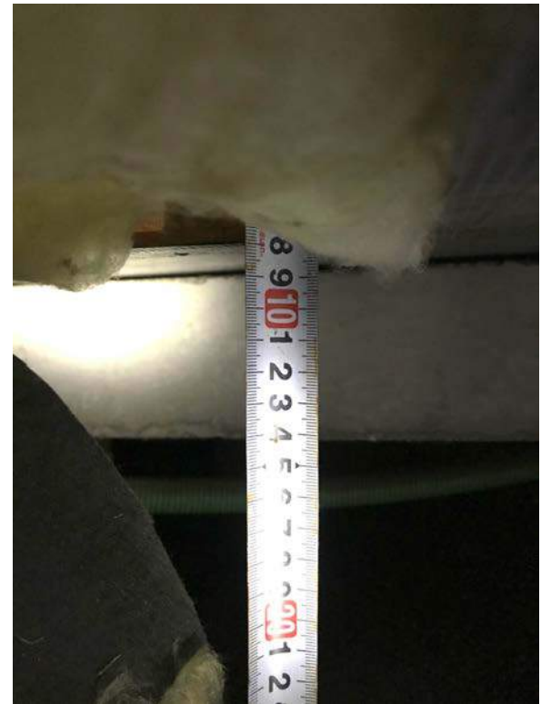
既存の床下断熱：GW厚80mm
